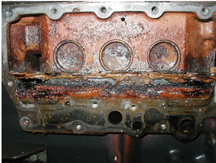
A 3 Crankcase in the area of the lubricating oil cooler housing
